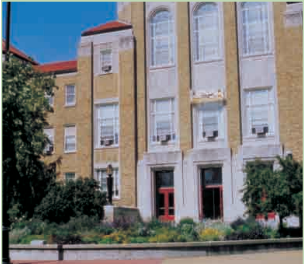
School officials installed more than 200 energy efficient windows and 1,229 lights in the high school. With the energy improvements at University City High School, officials expect energy savings to exceed $137,000, annually.
