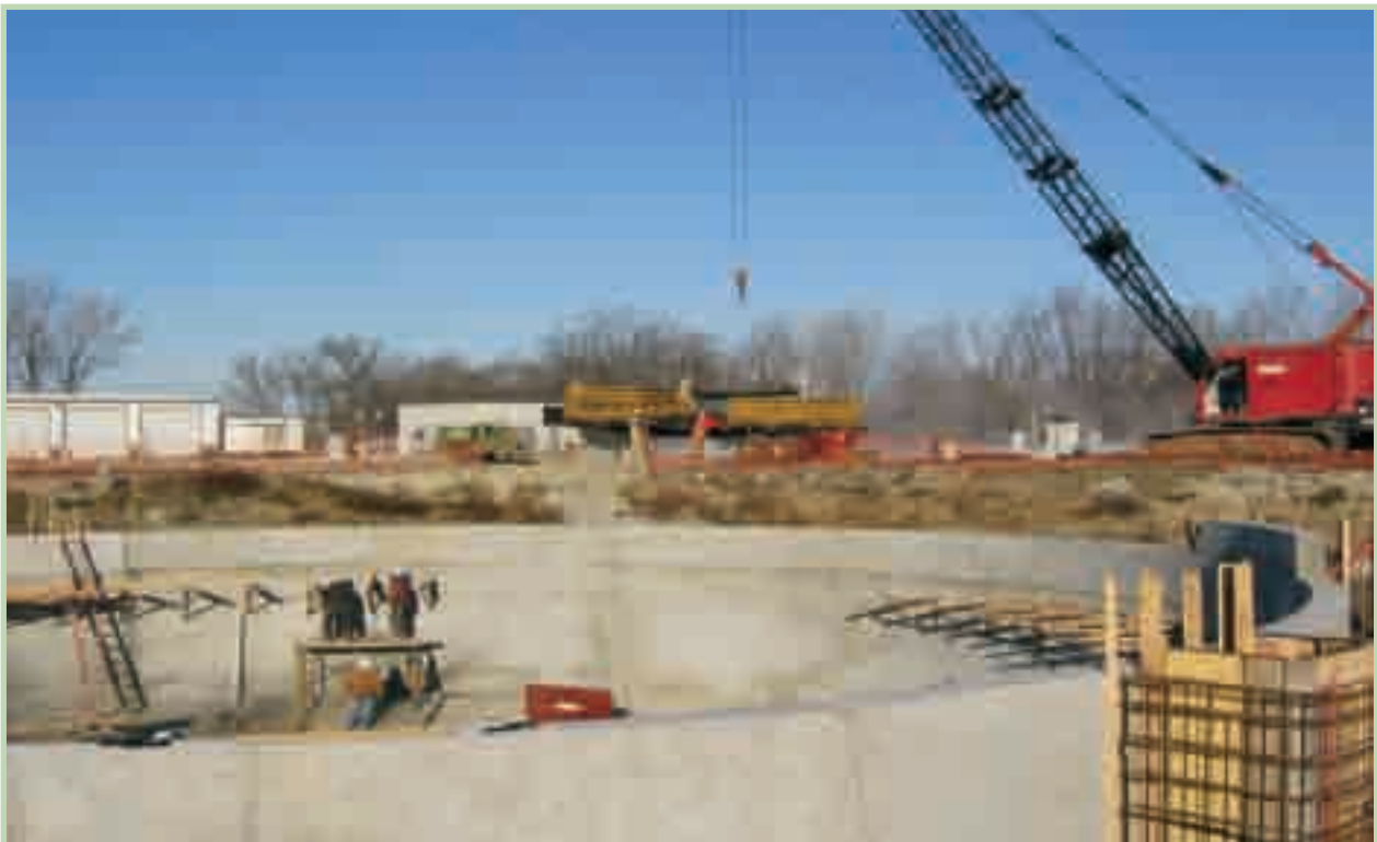
This clarifier, which is 50 feet in diameter, removes scum and sludge from the wastewater. The clarifier, under construction at the Trenton wastewater treatment plant, is designed for an average flow of 3 million gallons a day. Trenton's main plant, one of the largest treatment facilities in northwest Missouri, sits on five acres, but the entire complex covers 100 acres.
