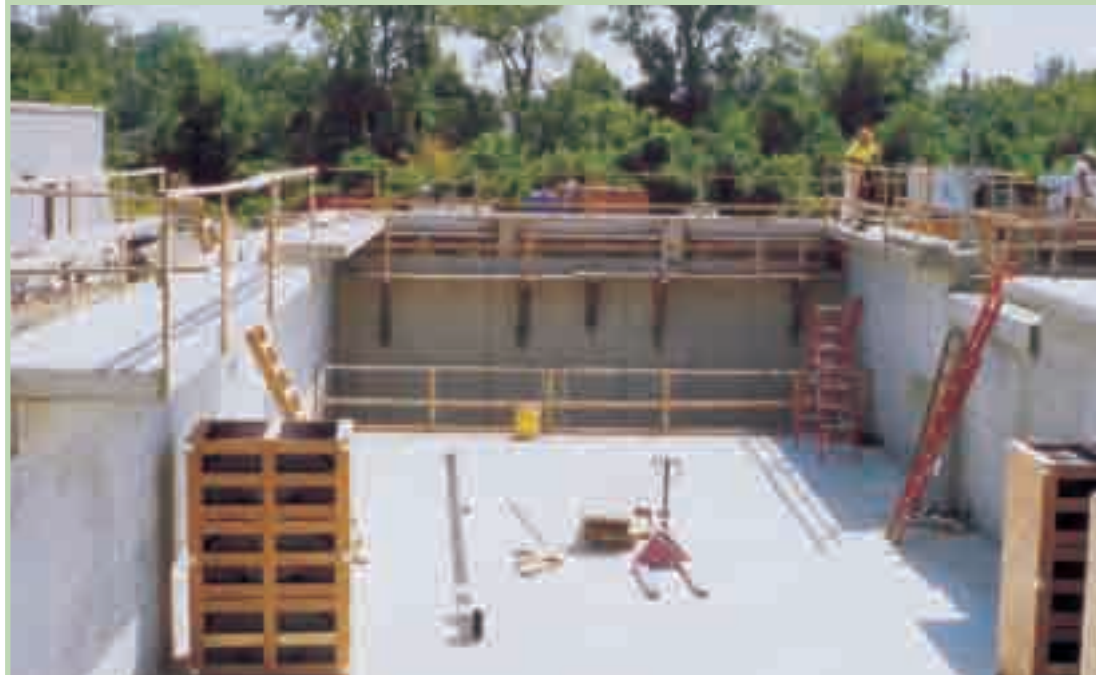
In this “cell” which is 100 feet by 30 feet and 22 feet deep, wastewater mixed with recycled sludge, rolls over and under a vertical loop and organics and other pollutants are removed. The vertical loop reactor, under construction at Washington’s wastewater treatment plant, is an innovative biological process in the treatment industry and will be the first operation of this type in Missouri.
