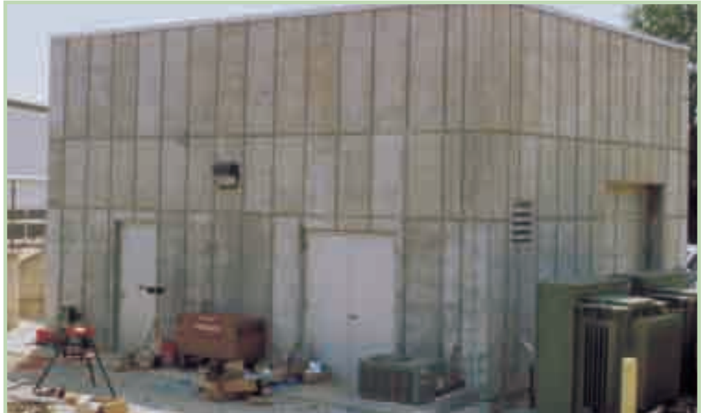
In 1997, Trenton officials received a $5 million loan from State Revolving Fund to build a new headworks system, which included this 6-pump lift station and other improvements, such as the installation of a grit removal system and upgrades to the collection system.
