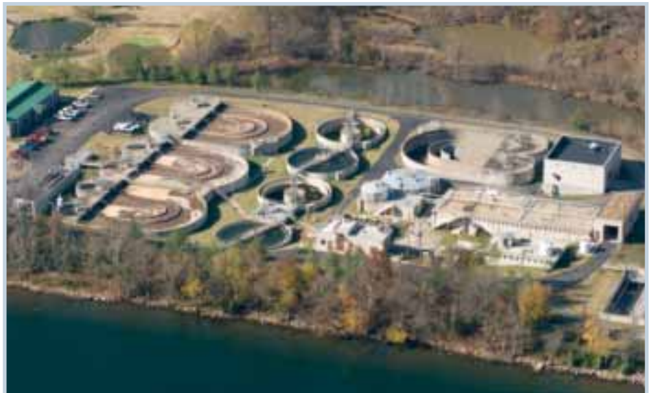
Since 1972, the Authority has issued bonds totaling more than $4.8 billion for environmental and infrastructure improvements, which includes the construction of wastewater treatment and public drinking water facilities. The facility pictured here is the Branson wastewater plant, which processes 5.3 million gallons a day.
