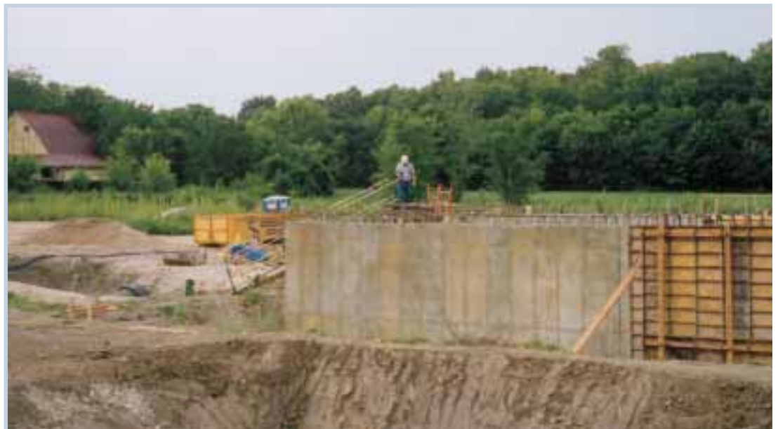
When completed, the UV (ultra violet-light) Building will be one part of a large improvement project at the Wentzville wastewater treatment plant, supported by a $19.4 million loan through the State Revolving Fund (SRF). City leaders stated by using the SRF they will realize an annual savings of $471,000.
