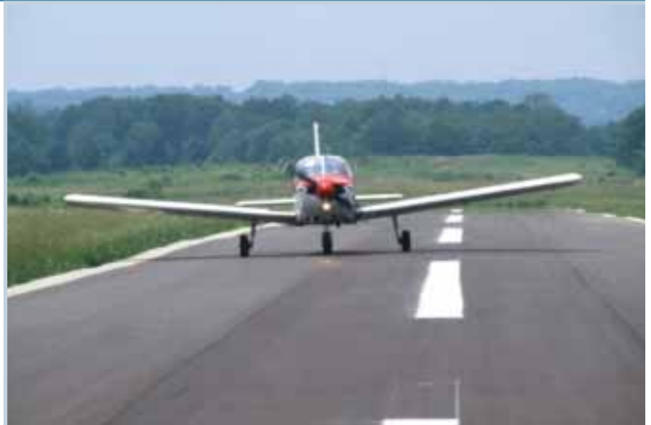
This 3,000-foot runway, taxi area and parking apron at the Rolla Downtown Airport were paved with 4,000 tons of Glasphalt, a mixture that included asphalt and 400 tons of recycled glass. In 1997, the airport, which is the first aviation facility in the United States to use Glasphalt, received $150,000 in assistance from EIERA's Market Development Program.
