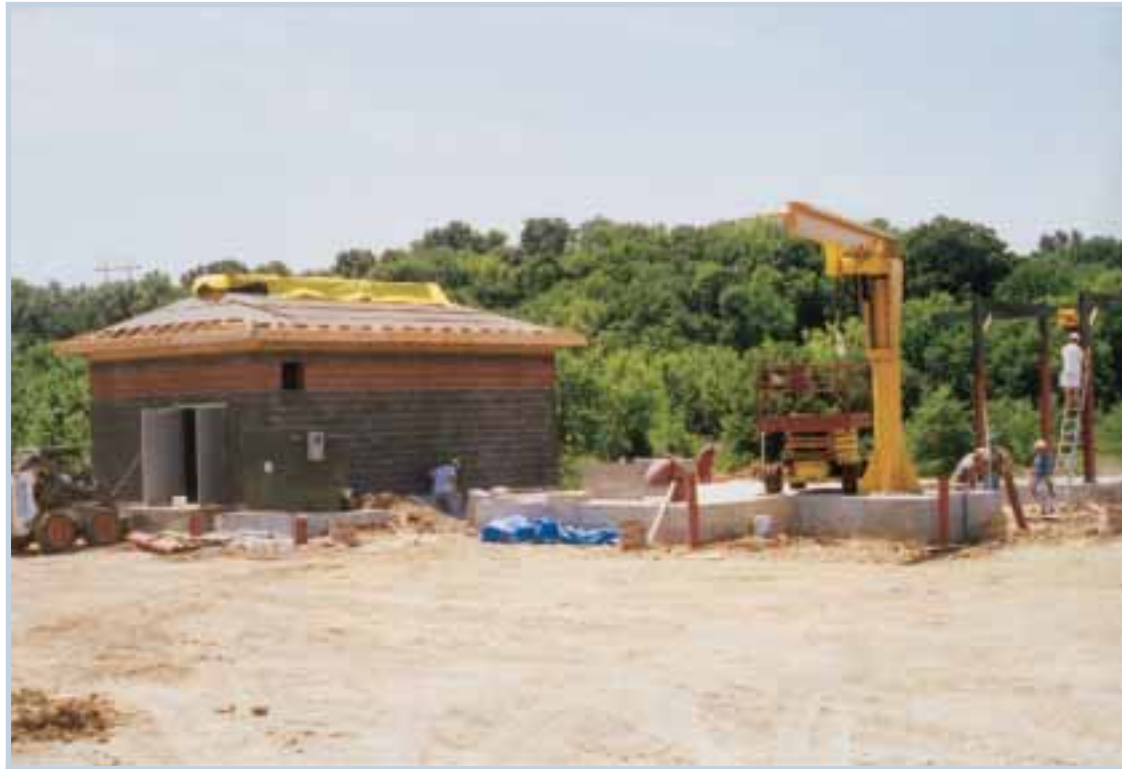
When completed, this $2 million pump station in Liberty will push 2 million gallons of wastewater daily to Kansas City to be treated. The pump station was one phase in an improvement project assisted by a $6.1 million loan from the State Revolving Fund.
