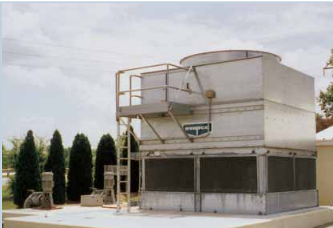
This 14-foot cooling tower, which weights more than 11,000 pounds and pumps 1,050 gallons of water per minute, was purchased with a $1.1 million loan from Missouri Energy Efficiency Leveraged Loan Fund. With several other energy improvements, school officials at Mineral Area College will save more than $96,000 annually.
