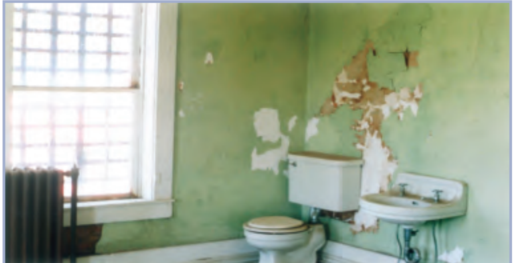
This toilet and washbasin, located on the second floor of the Linn County Jail, served the needs of women prisoners. The men's jail was secured behind a 500-pound steel door in the basement. The Linneus Museum and the Linn County Museum Association received financial assistance to remove lead paint, asbestos and other contaminants from the property.
