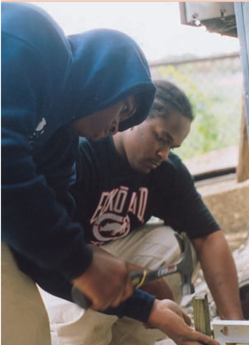
Robert Randle, 19, watches closely as Clarence Howard, 21, hammers a stud in place before concrete is poured. Randle and Howard are enrolled in YouthBuild St. Louis with 20 other young men and women. They learn carpentry and building skills at construction sites, while attending high school to earn their GED.
