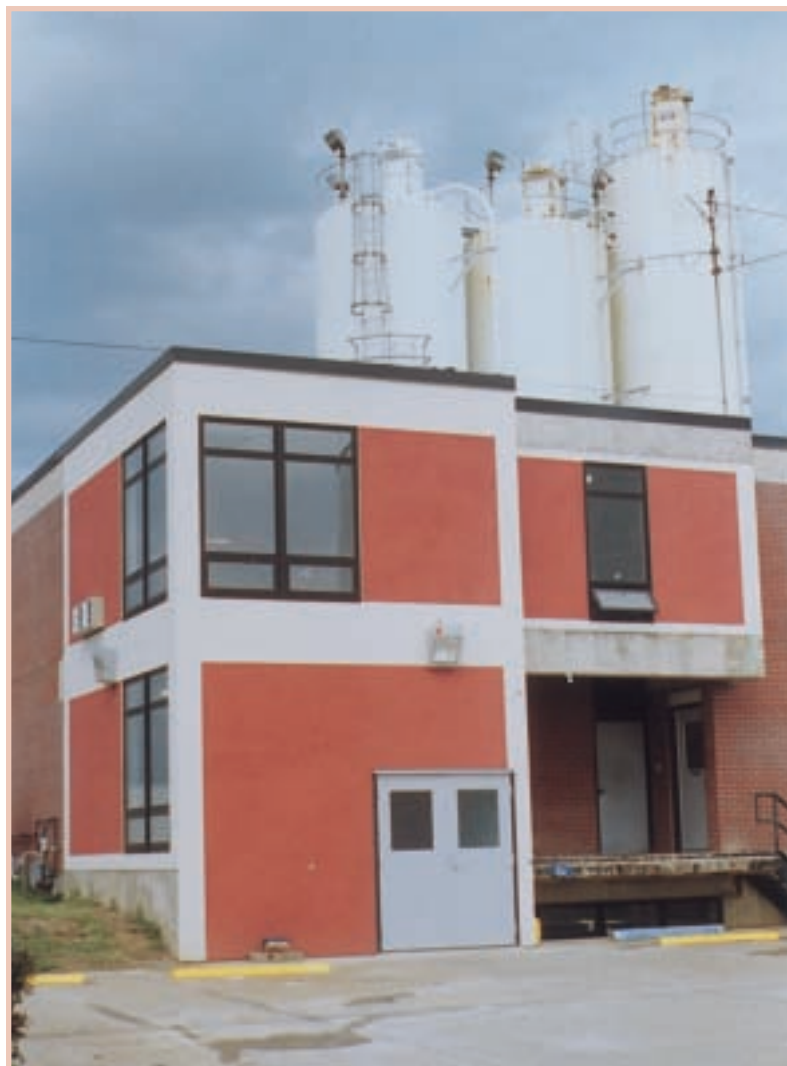
The Kirksville Water Plant, which employs eight workers, received a $1.8 million loan from the State Revolving Fund. The financial assistance provided equipment upgrades as well as construction improvements to the exterior and interior areas of the building. The plant serves Kirksville and several nearby communities.
